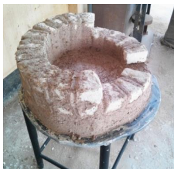
Plate 10: Laying second row of bricks
