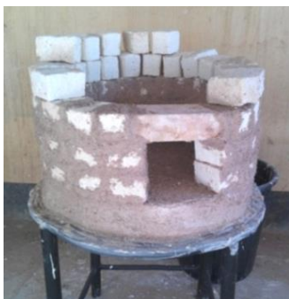
Plate 11: Third & fourth layer of bricks
