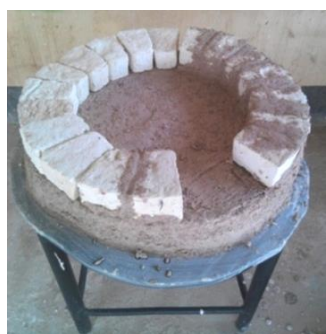
Plate 9: Laying first row of bricks
