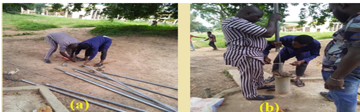
Figure 4: Repair and Assembling of (a) New High-durability Galvanized Pipes (b) Cylinder Insertion into Borehole
