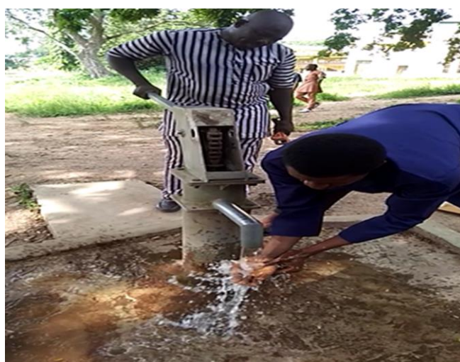
Figure 5: Testing of the Repaired Hand Pump
