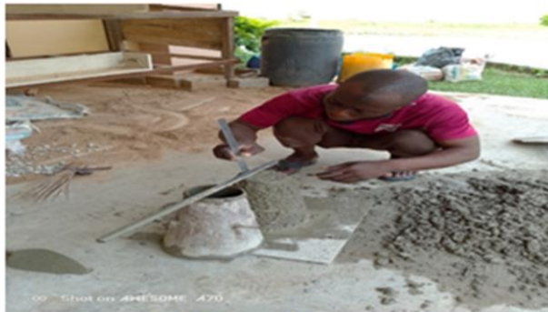
(a) Slump Test
